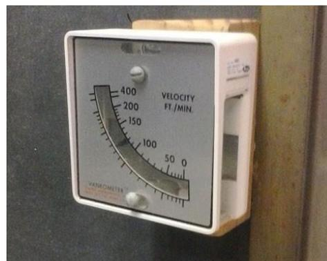
Figure 2. ECS hood Vaneometer. Note airflow reading above 100 LFM (arrow).
