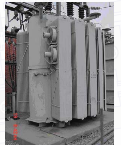
FIGURE 4 - 10 MVA Transformer
