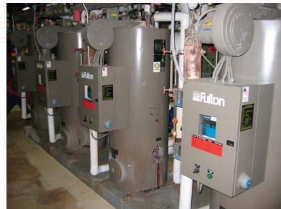
Building 41 Steam Boilers
