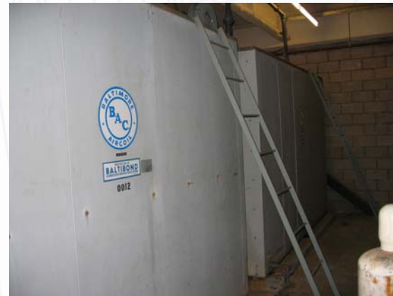
Building 83 TES Units
