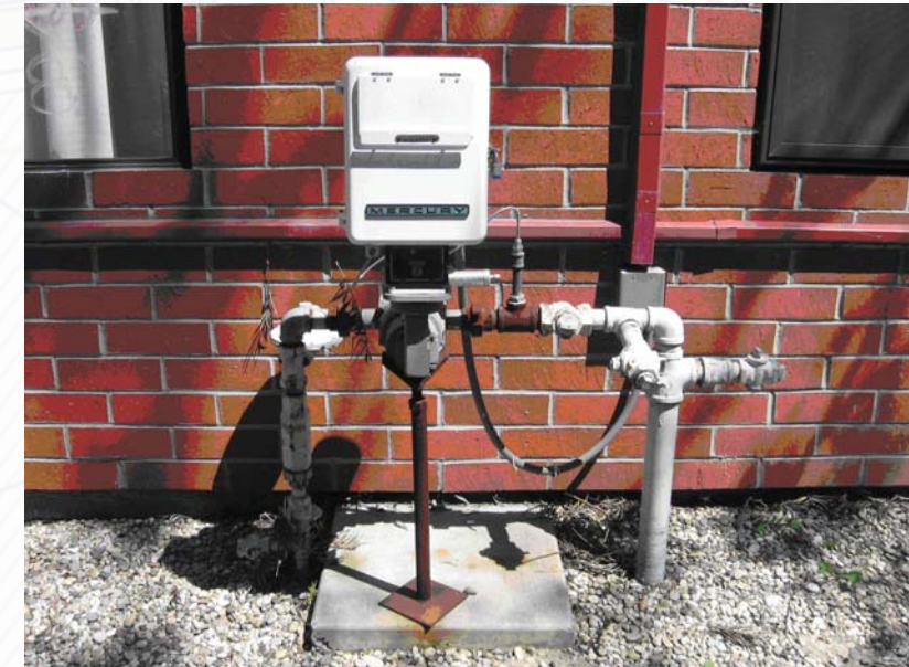
FIGURE 1 - Typical Natural Gas Meter
