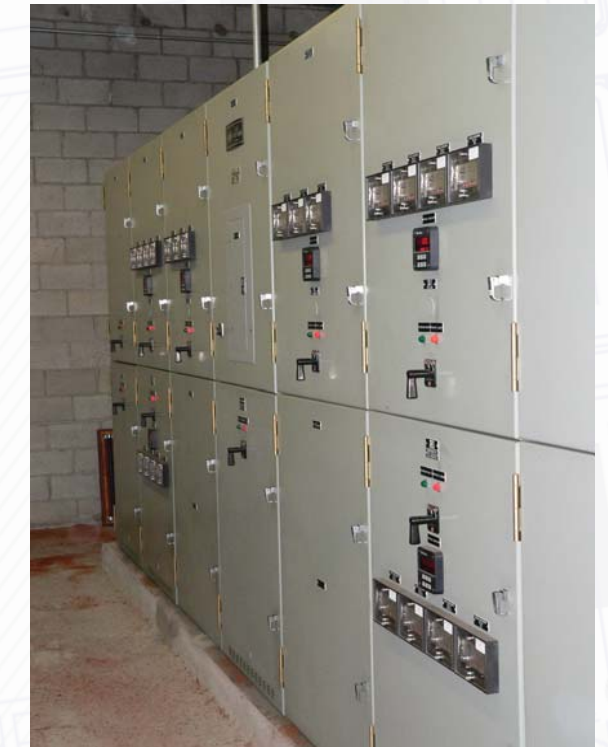
FIGURE 2 - Main 12 kV South Switchgear
