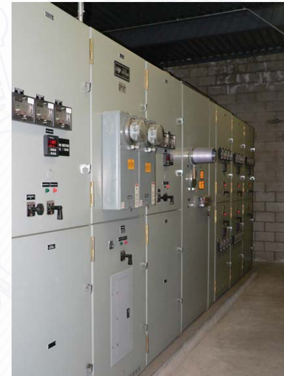
FIGURE 1 - Main 12 kV North Switchgear
