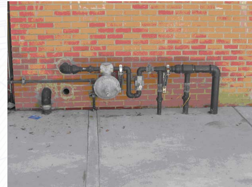
FIGURE 1 - Typical Natural Gas Pressure Regulator
