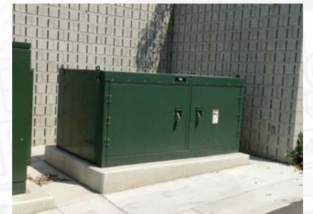
FIGURE 3 - 15 kV Selector Switch - Typical
