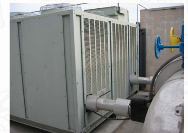
Building 73 Chiller Connection
