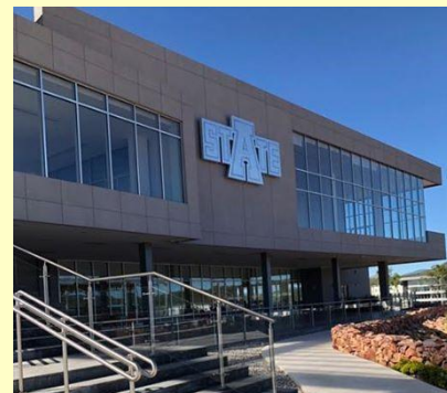
Outside of the Main Campus Building
