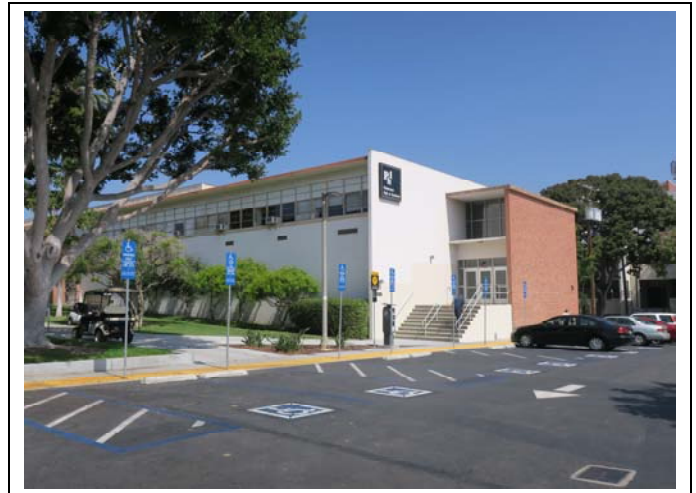
Image 5. South and east façades, view northwest (ARG, 2019)
