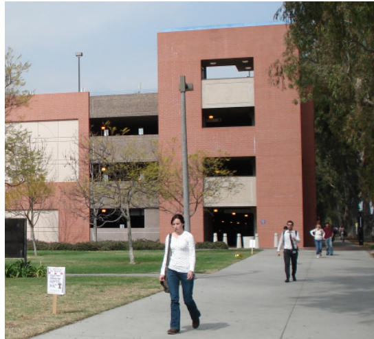
Parking Structure No. 1
