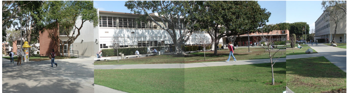
Peterson Hall I and II, in the Liberal Arts area of campus, are to be demolished and replaced.
