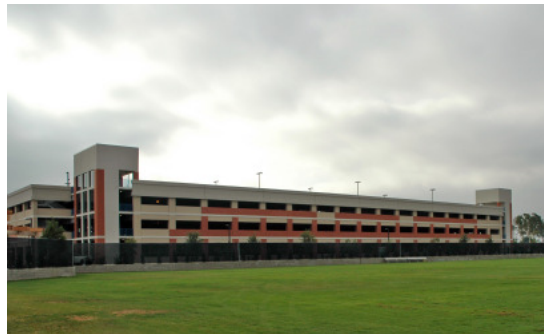
Parking Structure No. 2
