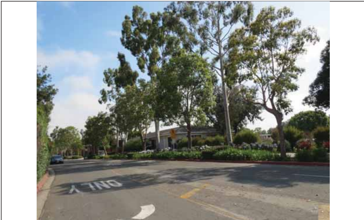
Figure 18. North and east elevations from Earn Warren Drive, (IMG_3478)
