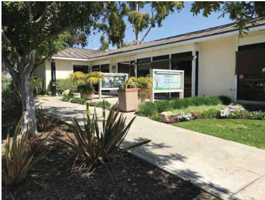
Figure 7. Landscaping with exposed soils along the western façade of the HRL Office building. Photo taken from the southeast corner of HRL Office building. View to the northeast.
