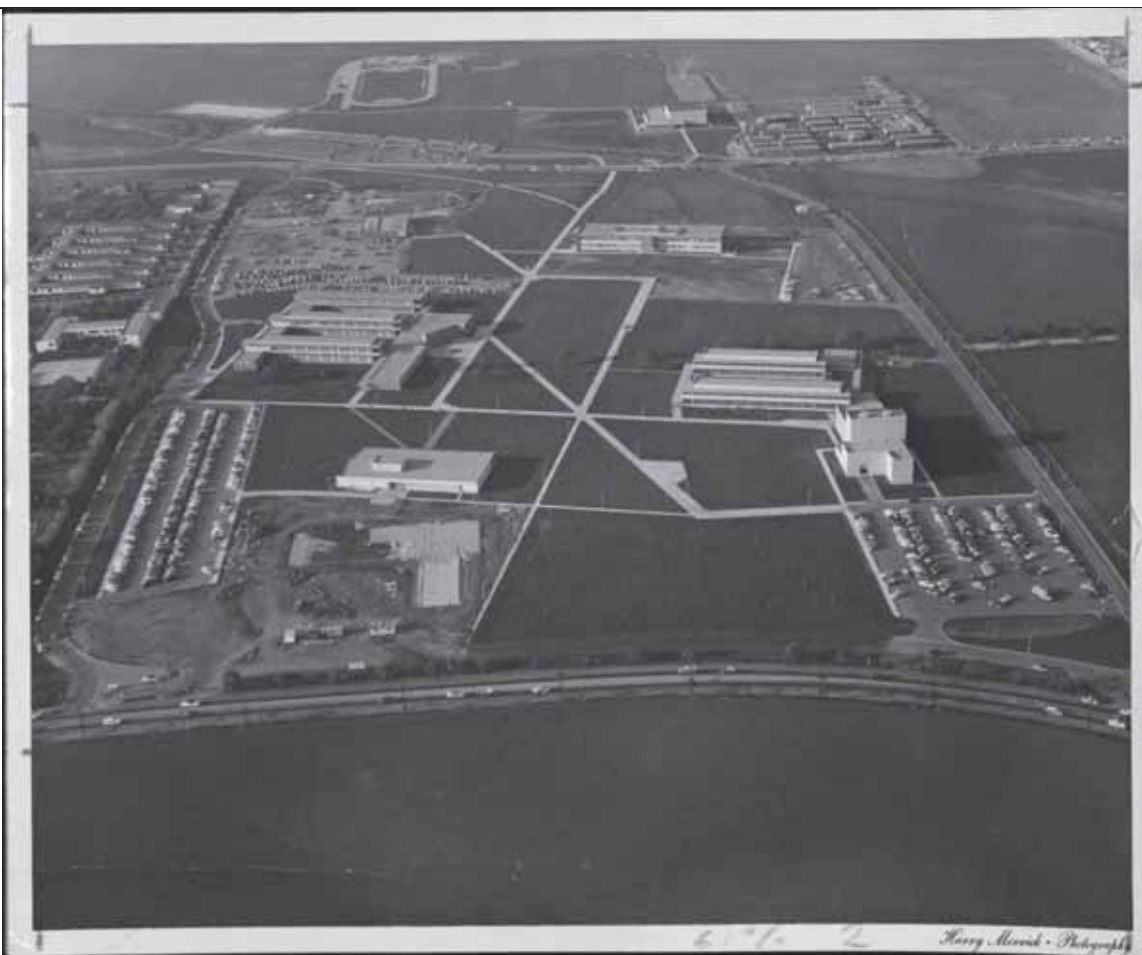
Figure 7. Upper Campus, looking north to lower campus, administration building under construction on foreground, 1955 (CSULB Special Collections)
