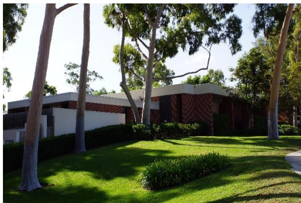
Figure 2-4b Northwest Elevation Looking Southeast
