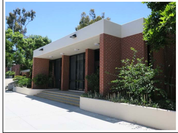
Figure 18. Building G, Hillside Office/ Commons, rear (east) elevation, view southwest (ARG, 2019).
