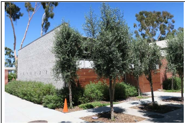
Figure 23. Building H/Hillside Dining, west elevation, view northeast. Note dining patio addition in foreground (ARG, 2019).
