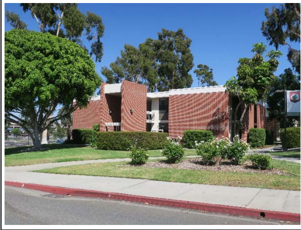
Figure 15. Building F as seen from Earl Warren Drive, view northeast (ARG, 2019).
