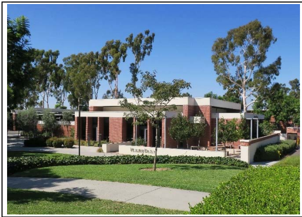
Figure 21. Building H/Hillside Dining, primary (south) elevation, view northwest (ARG, 2019).
