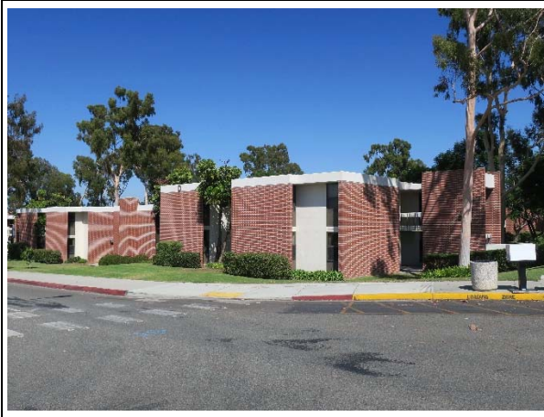
Figure 9. Building D as seen from Earl Warren Drive, view northeast (ARG, 2019).
