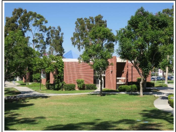
Figure 12. Building E as seen from interior landscape, view northeast (ARG, 2019).
