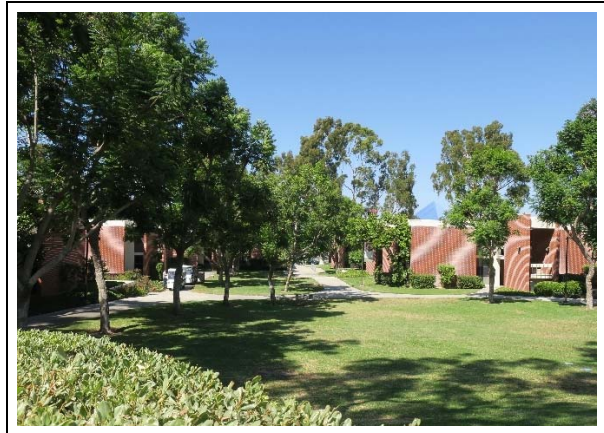
Figure 26. Landscape, view northeast, with Buildings D and E at left and right, respectively (ARG, 2019).
