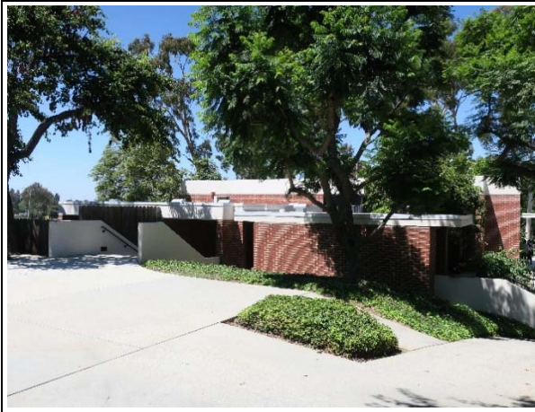
Figure 19. Building G, Hillside Office/ Commons, south elevation, view north (ARG, 2019).
