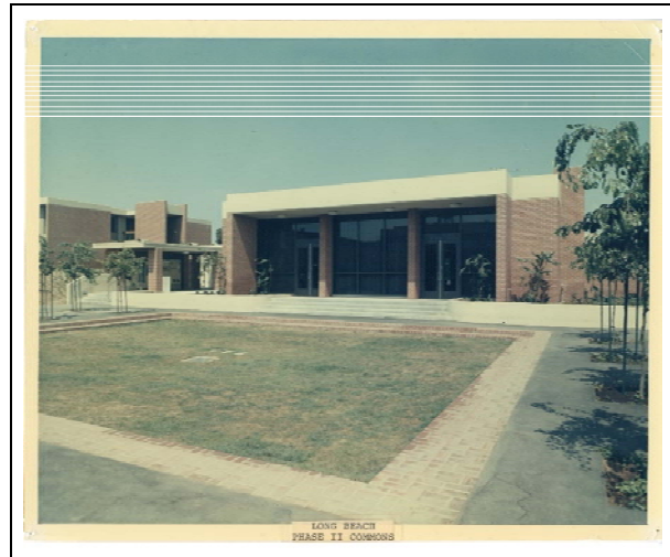
Figure 34. Building G, Commons (1972), view west. Note sunken plaza in foreground, which has since been removed (CSULB Library Special Collections and University Archives).
