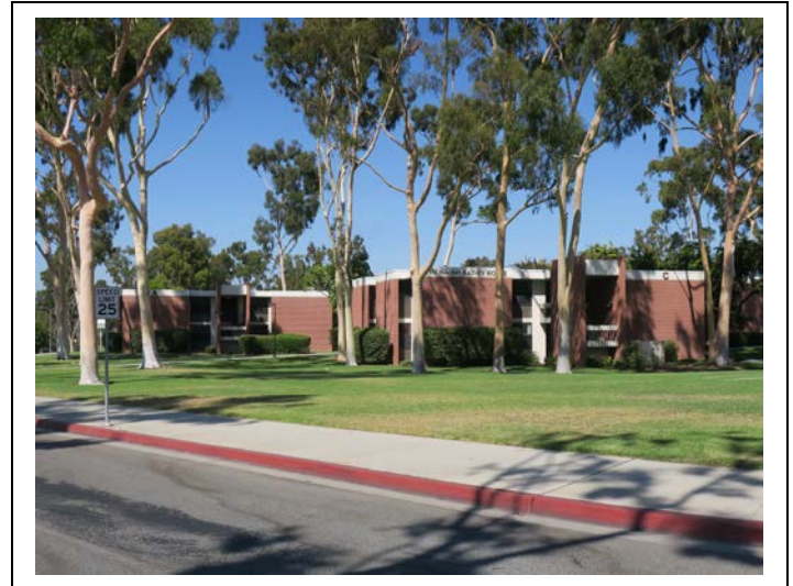
Image 5. Hillside College setting, view northeast (ARG, 2019).
