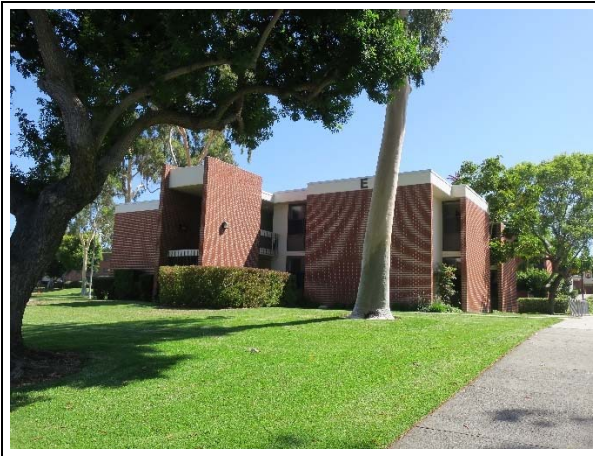
Figure 11. Building E as seen from Parking Lot G4, view south (ARG, 2019).
