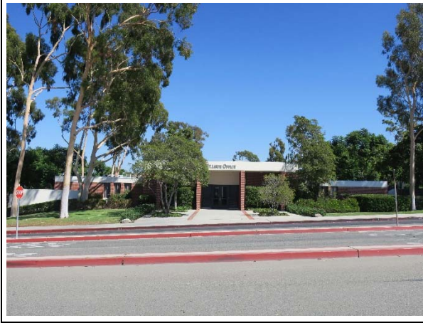
Figure 17. Building G, Hillside Office/ Commons from Earl Warren Drive, view southeast (ARG, 2019).
