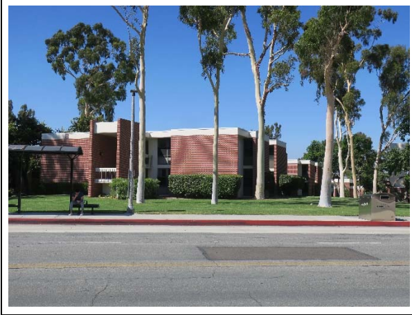
Figure 7. Building B as seen from Beach Drive, view north (ARG, 2019).
