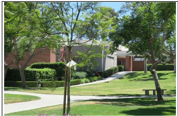
Figure 24. Building H/Hillside Dining, view south. Note addition with enameled panels in foreground (ARG, 2019).
