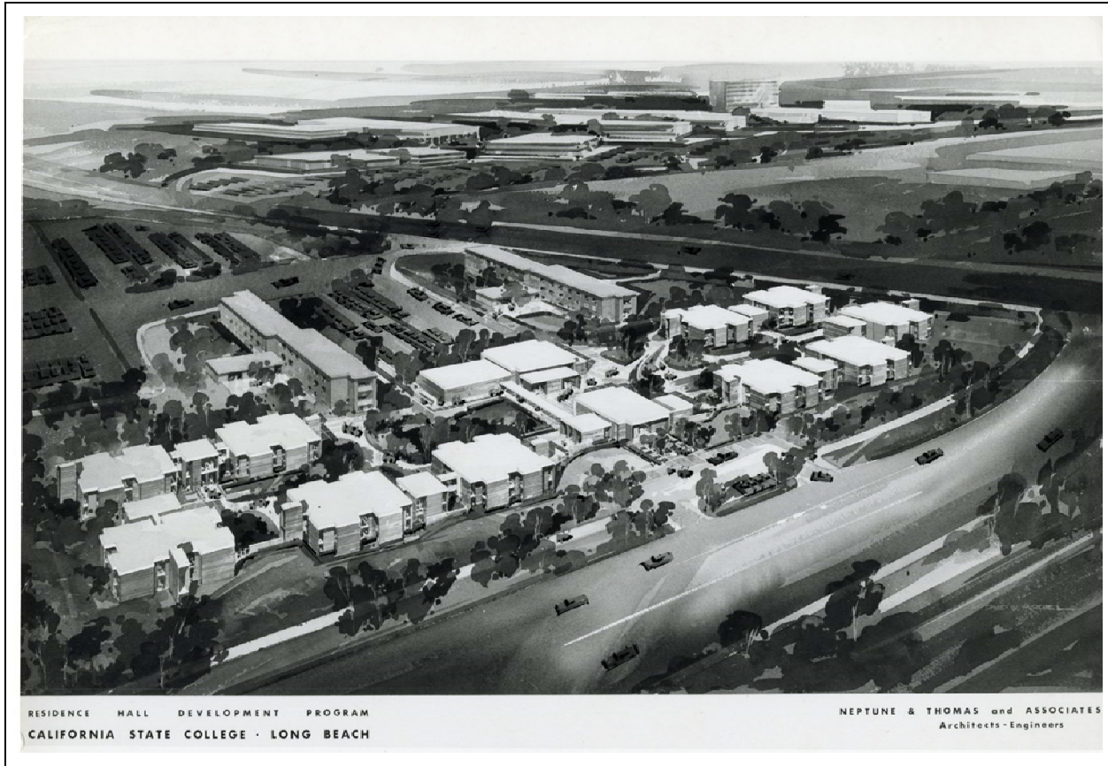
Figure 32. Rendering of Residence Hall Development Program Phase II (ca. 1966), Neptune and Thomas & Associates. The complex was re-named Hillside College (CSULB Library Special Collections and University Archives).
