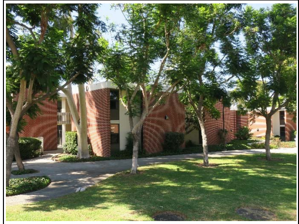
Figure 10. Building D as seen from interior landscape, view north (ARG, 2019).
