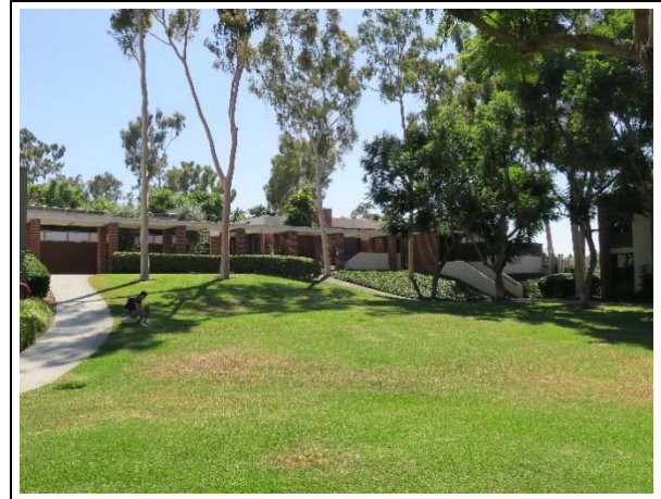
Figure 20. Building G, Hillside Office/ Commons, north elevation and breezeway, view southwest (ARG, 2019).
