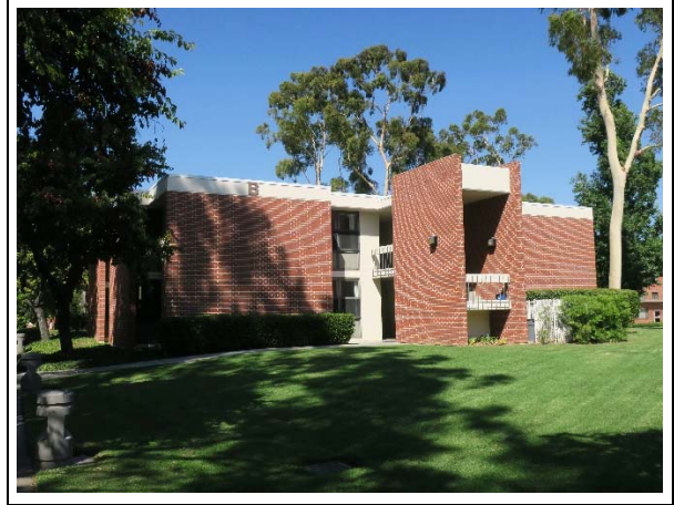
Figure 8. Building B, view northeast (ARG, 2019).
