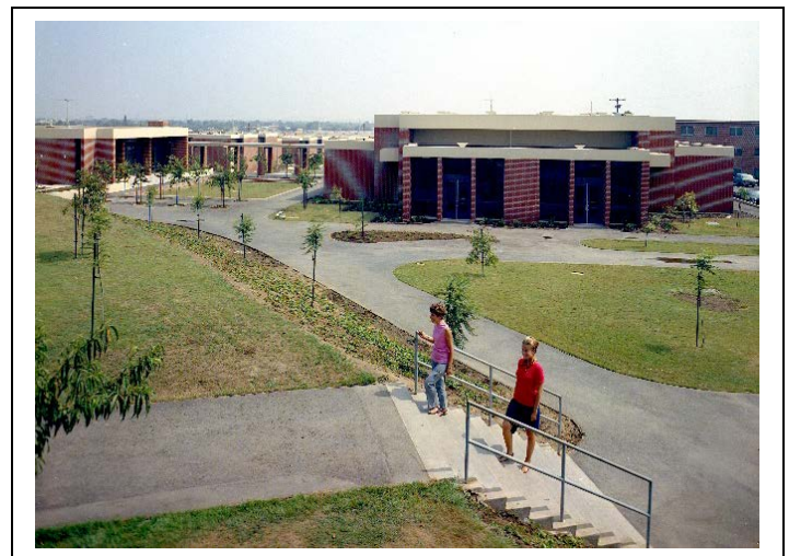
Image 7. Residence Hall Development Program Phase II, 1969 (CSULB Library Special Collections and University Archives).
