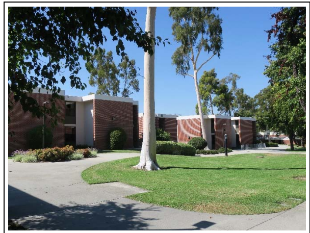
Figure 6. Building A as seen from interior landscape, view north (ARG, 2019).
