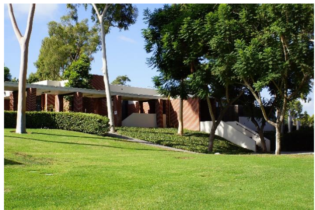
Figure 2-4c Northeast Elevation Featuring Covered Walkway Connecting to Hillside College Dining Hall (left), Looking Southwest
