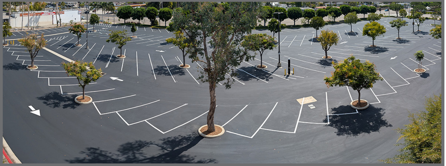
Asphalt overlay and restripe of Lot G13
