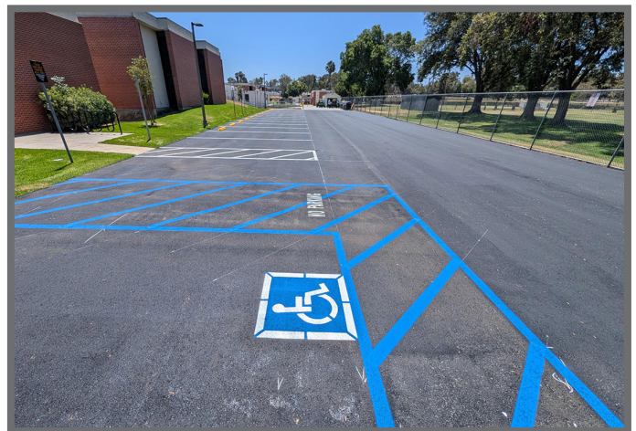
Asphalt overlay and restripe of the Parkside Commons parking area
