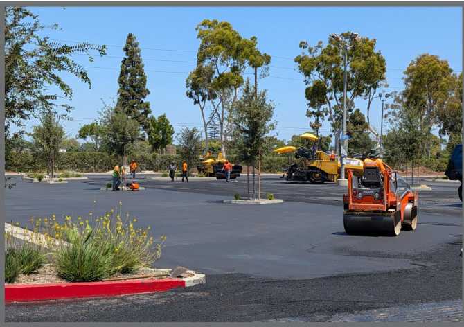
Asphalt overlay and restripe of Lot G9
