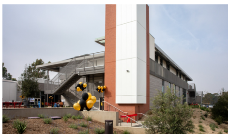
Hillside Service Center
