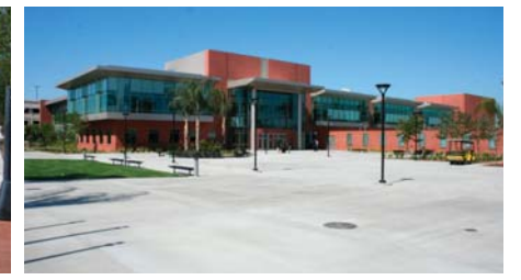
2. Brick with Concrete Bands
