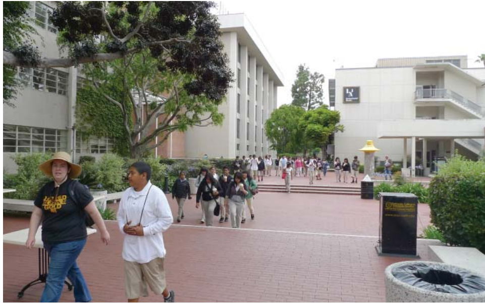
Major pedestrian route through depressed courtyard. Circulation issues for those with disabilities.
