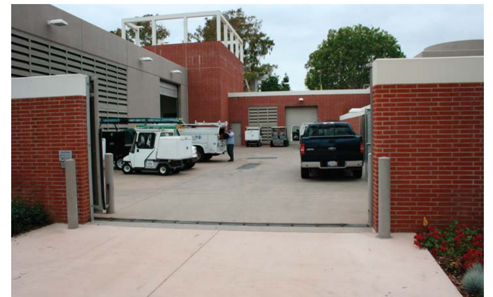
Campus Central Plant- Service and Utilities
