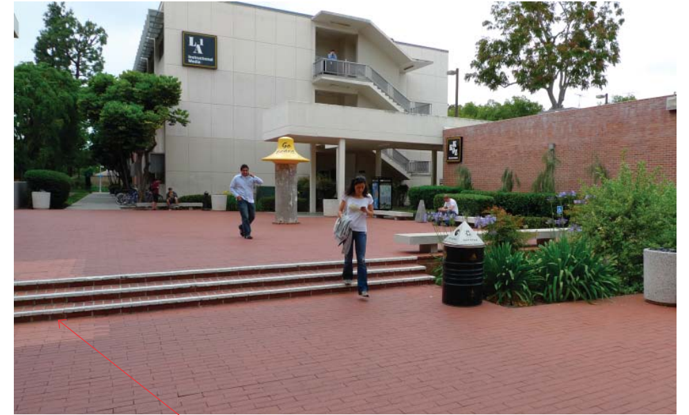
Areas in need of repair.
