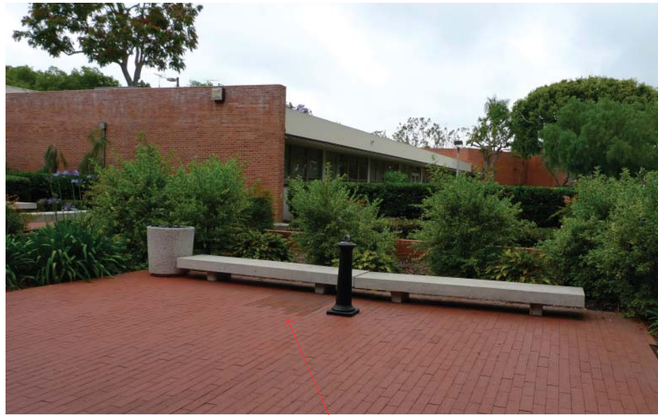
Areas in need of repair.
