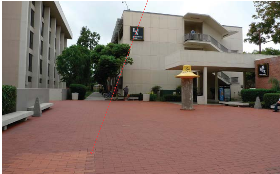
Areas in need of repair.
