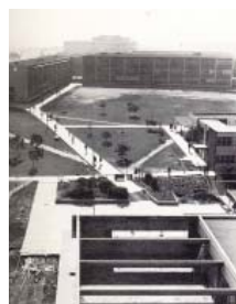
Construction on the new Cafeteria Addition
