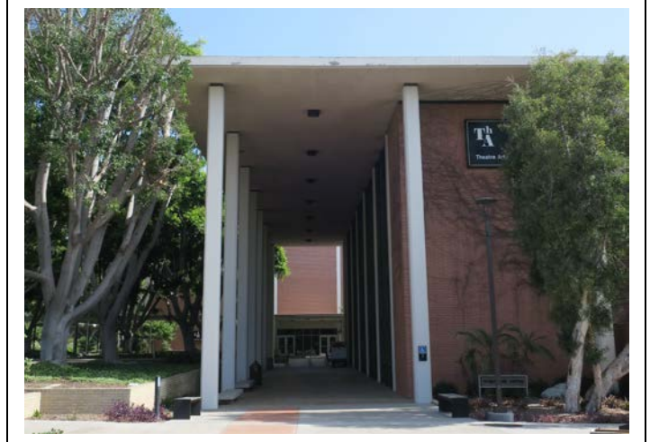
Image 3. South elevation, detail of colonnade, view north (ARG, 2019)
