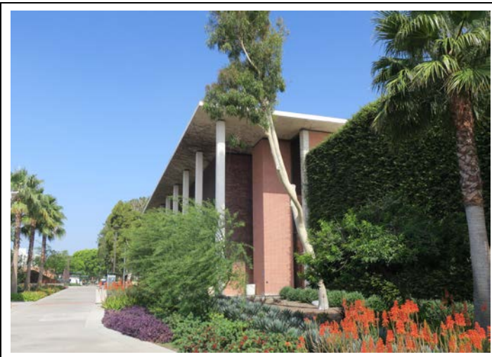
Image 4. South and east elevations, view northwest (ARG, 2019)
