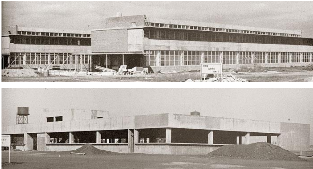
The Fine Arts Unit (top) and Library (bottom – now Academic Services) were among the first permanent buildings to be constructed at the CSULB campus in the mid-1950s (CSULB)
