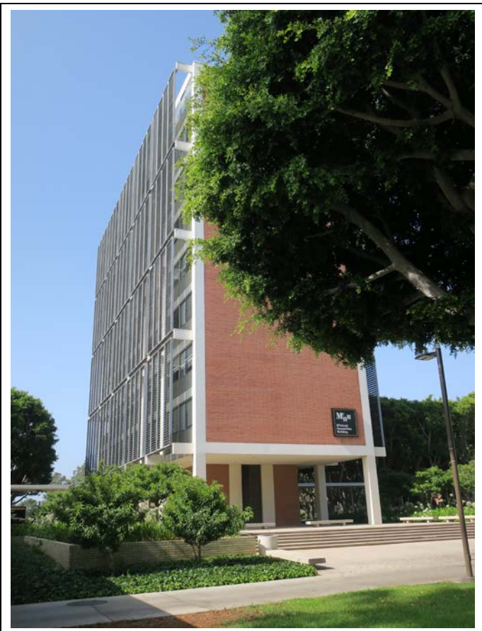
Image 4. North and east elevations, view southwest (ARG, 2019)
