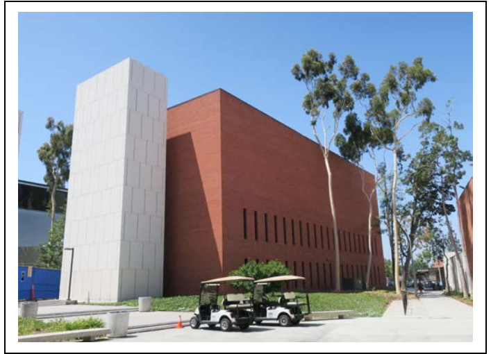
Image 3. North elevation, view southwest (ARG, 2019)
