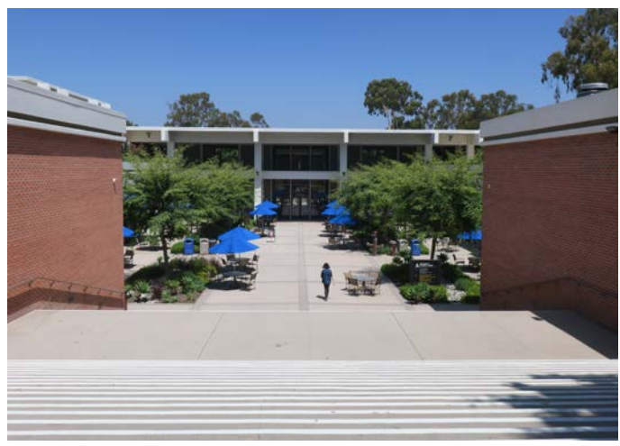
Image 4. South elevation, view northeast (ARG, 2019)
