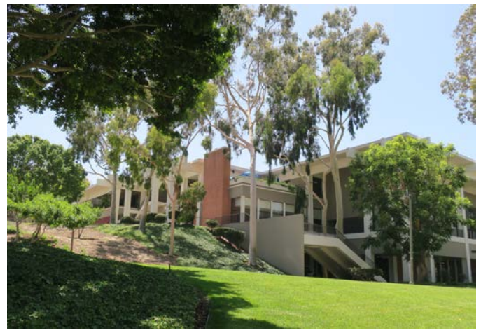
Image 3. North and east elevations, view southwest (ARG, 2019)
