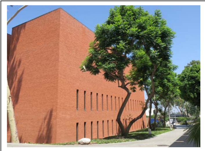
Image 4. South elevation, view northeast (ARG, 2019)
