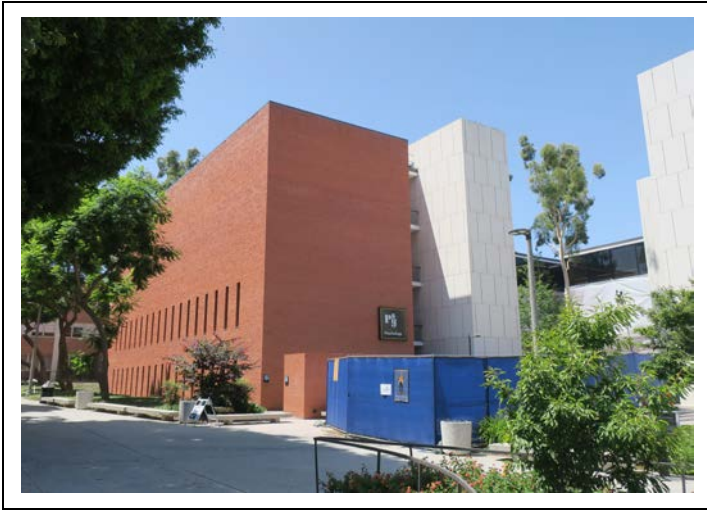
Image 2. East elevation, view southwest (ARG, 2019)
