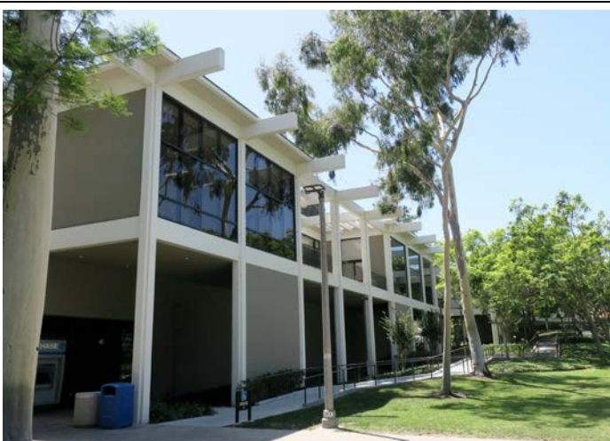
Image 6. West elevation, view southeast. This portion of the building dates to 1998 (ARG, 2019)
