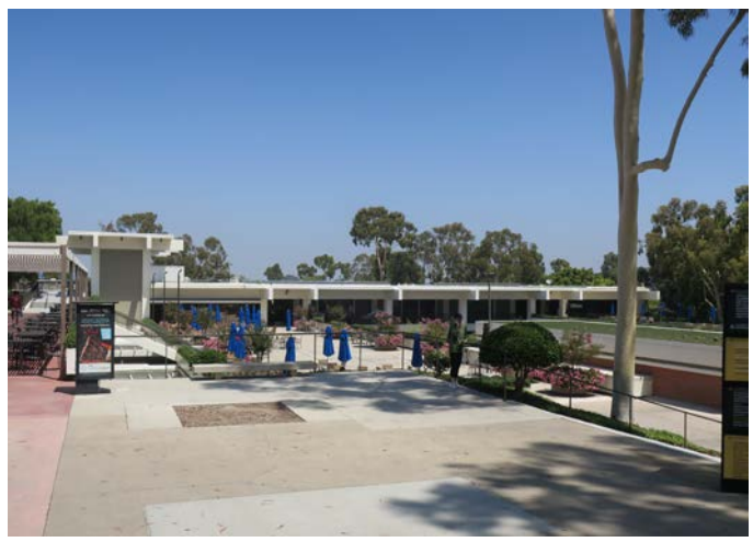
Image 5. South elevation, detail of sunken forecourt, view north (ARG, 2019)
