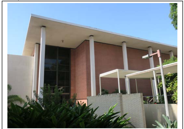
Image 5. North elevation, view southwest (ARG, 2019)
