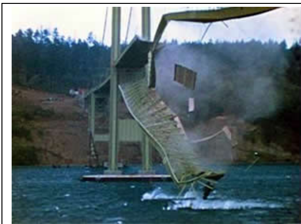
Film depicting the collapse of the Tacoma Narrows Bridge due to forced oscillatory motion. Movie from youtube . Click on image to view the movie.
