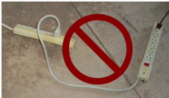
Not OK: daisy chain with 2 power strips
