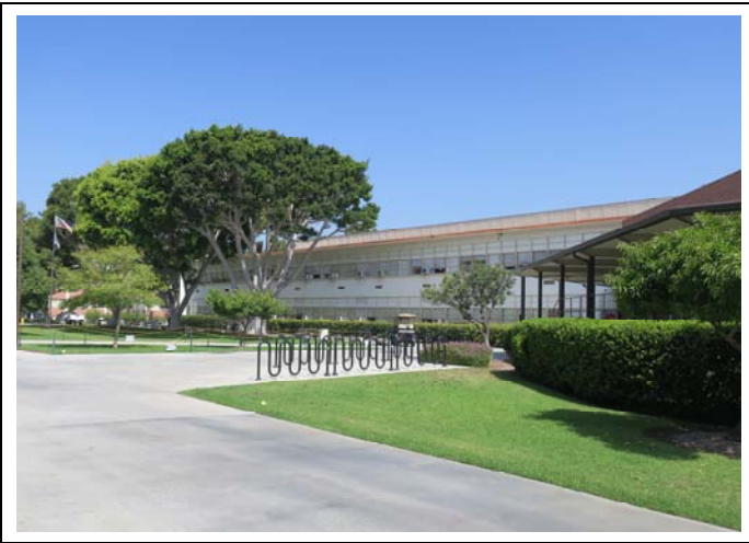
Image 2. South façade, view northwest (ARG, 2019)
