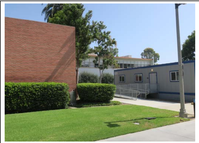
Image 4. South façade, view northeast (ARG, 2019)
