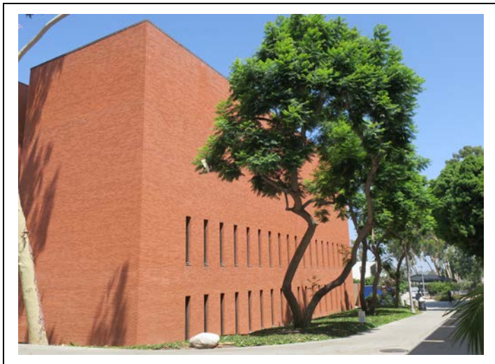
Image 4. South elevation, view northeast (ARG, 2019)
