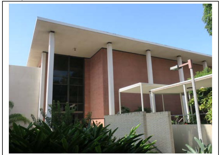
Image 5. North elevation, view southwest (ARG, 2019)
