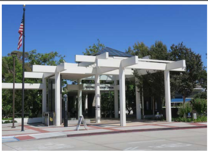
Image 7. Entrance canopy at west of building, view southeast. This portion of the building dates to 1998 (ARG, 2019)
