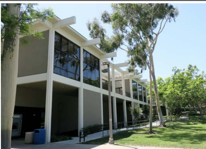
Image 6. West elevation, view southeast. This portion of the building dates to 1998 (ARG, 2019)
