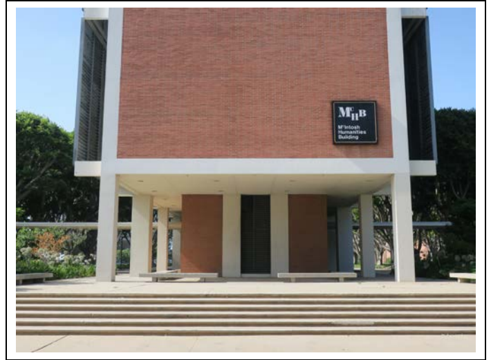
Image 3. Detail of north elevation, view south. Note recessed ground story and shallow plinth (ARG, 2019)
