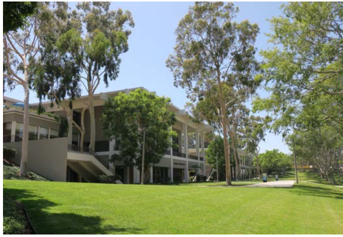
Image 2. North elevation, view southwest (ARG, 2019)
