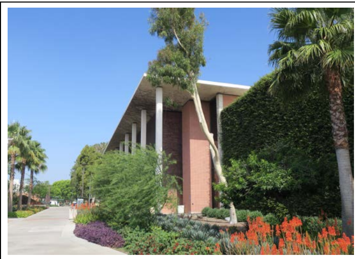
Image 4. South and east elevations, view northwest (ARG, 2019)
