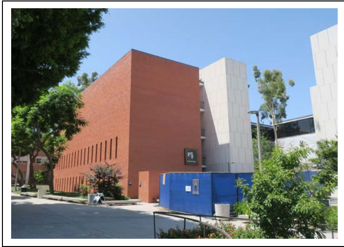
Image 2. East elevation, view southwest (ARG, 2019)
